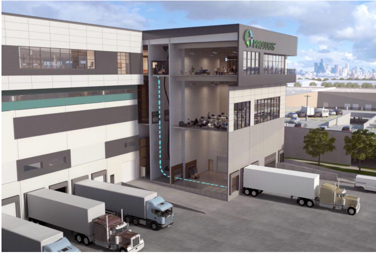
Prologis Georgetown Crossroads, as shown in this rendering, includes freight elevators with forklift access exclusively serving the third floor. PHOTO: STUDIO 216/PROLOGIS
