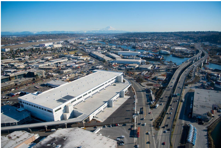
Prologis Georgetown Crossroads, a three-floor 590,000 square-foot industrial warehouse in Seattle. PHOTO: WOODY WELCH/PROLOGIS
